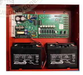
Unit rigid mounted to wall fixture with five (5) 1/4"x 3/4" wood screws. Washers were used in additon to the wood screw at each corner.
