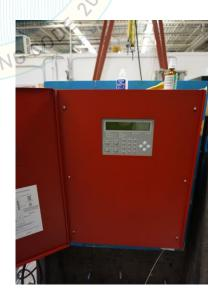
Unit rigid mounted to wall fixture with five (5) 1/4"x 3/4" wood screws. Washers were used in addition to the wood screw at each corner.
