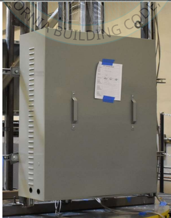
Overall view of UUT-02
