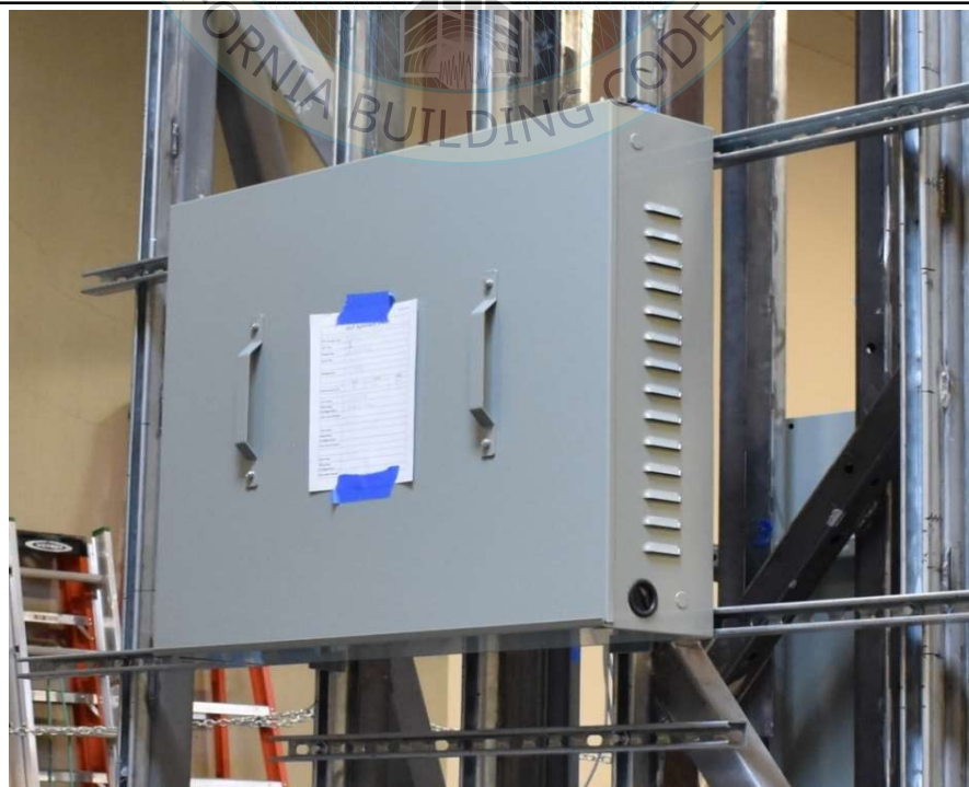
Overall view of UUT-01
