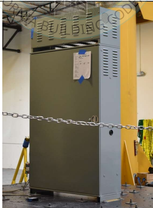
Overall view of UUT-03
