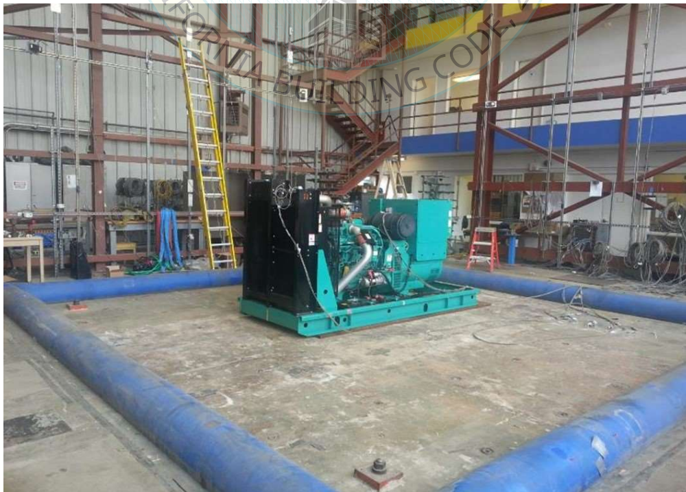
All units were filled with contents and maintained structural integrity and functionality after AC-156 test.
