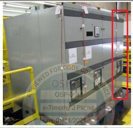
Manufacturer: CaterpillarTest Location: Wyle Laboratory, Inc.Product Line: Low Voltage Paralleling SwitchgearReport Number: 71152R13Matrix Identification: Magnum DS-3200UUT No. in Test Report: UUT-10
