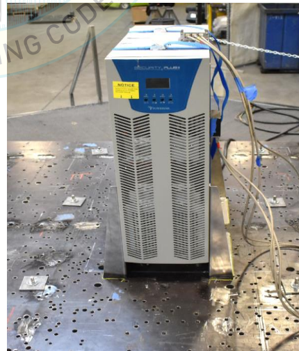
Figure 2. Front view of UUT1
