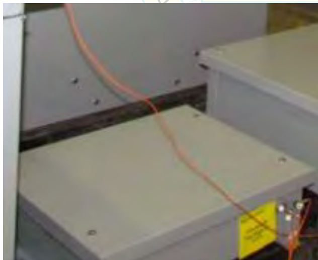
UUT-5 overall view.
