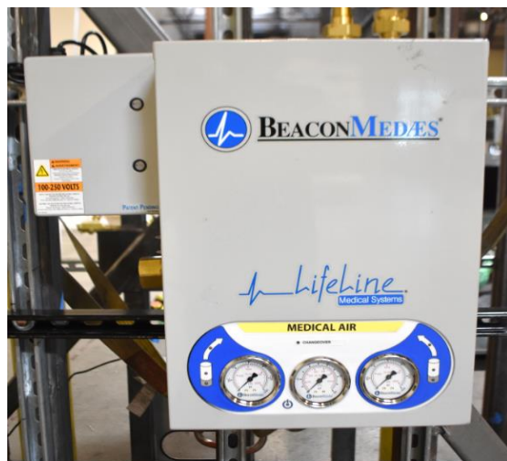
Figure 1. Overall exterior view of UUT-1
