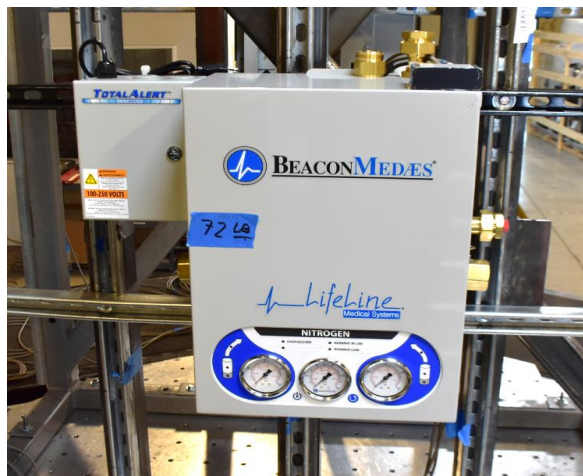
Figure 1. Overall exterior view of UUT-2
