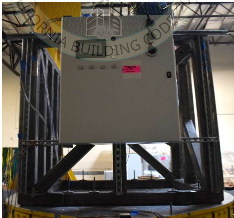
Figure 1. Overall view of UUT-23a
