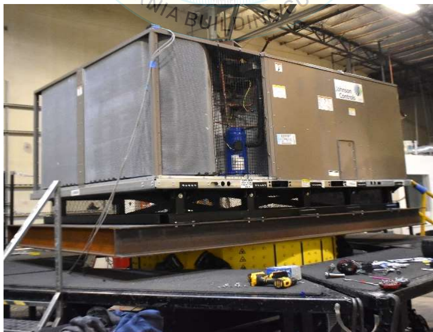
Overall view of UUT-02
