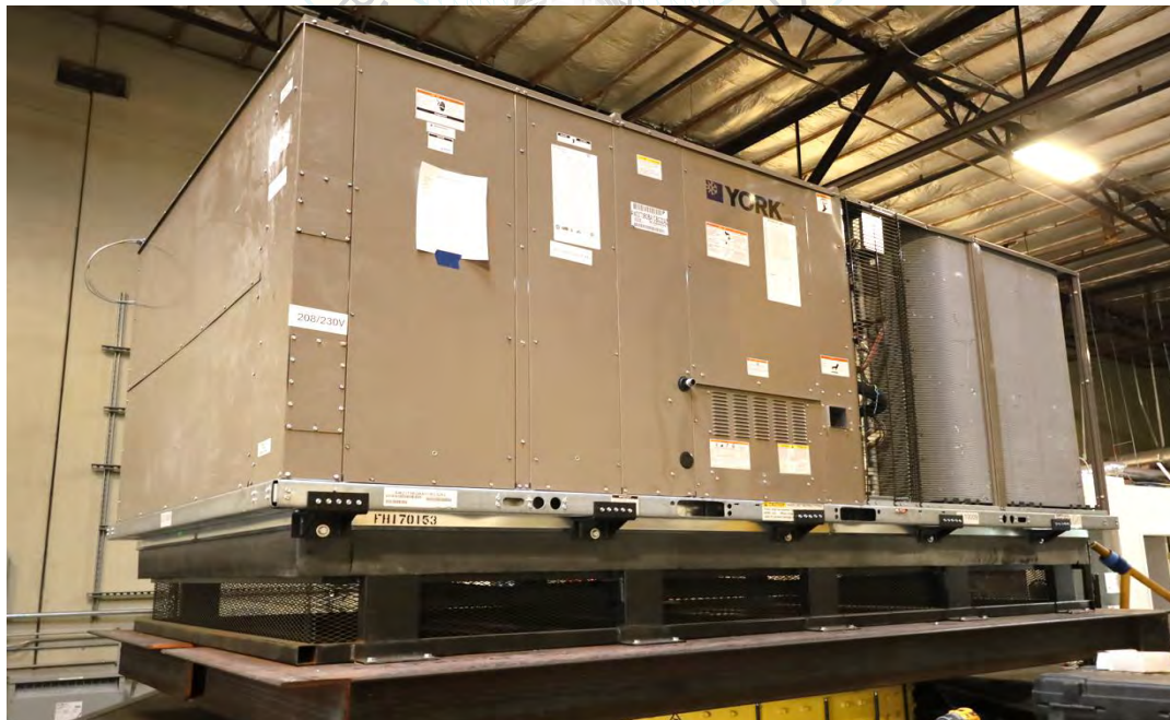
Overall view of UUT-08
