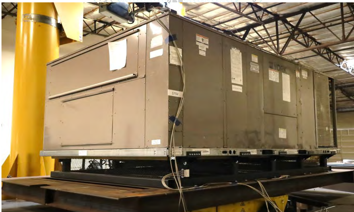
Overall view of UUT-05
