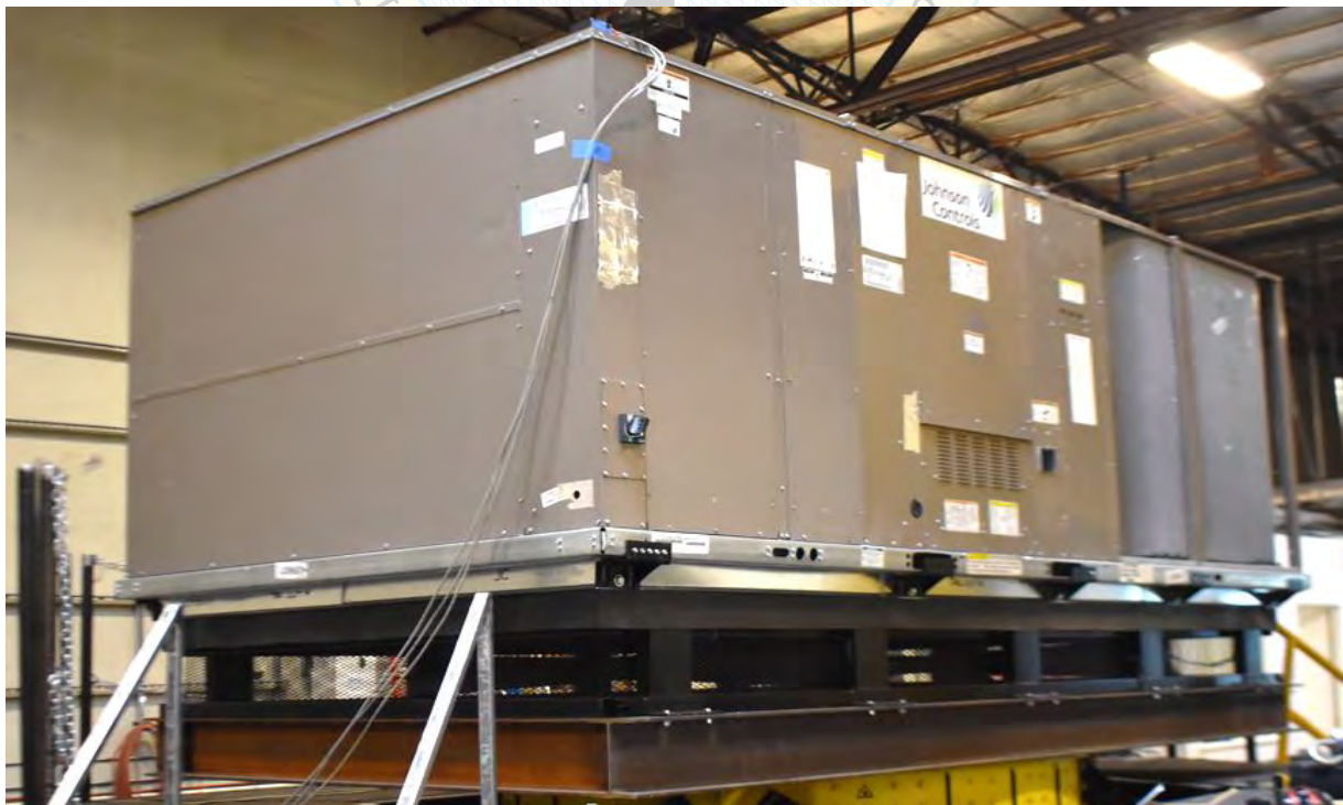
Overall view of UUT-04
