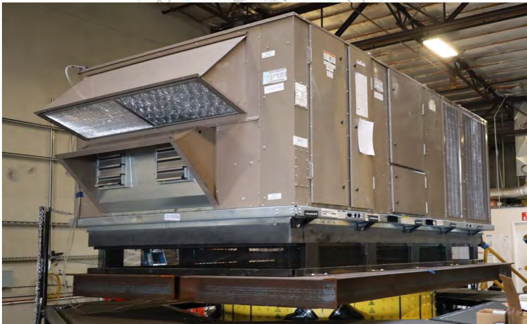
Overall view of UUT-06
