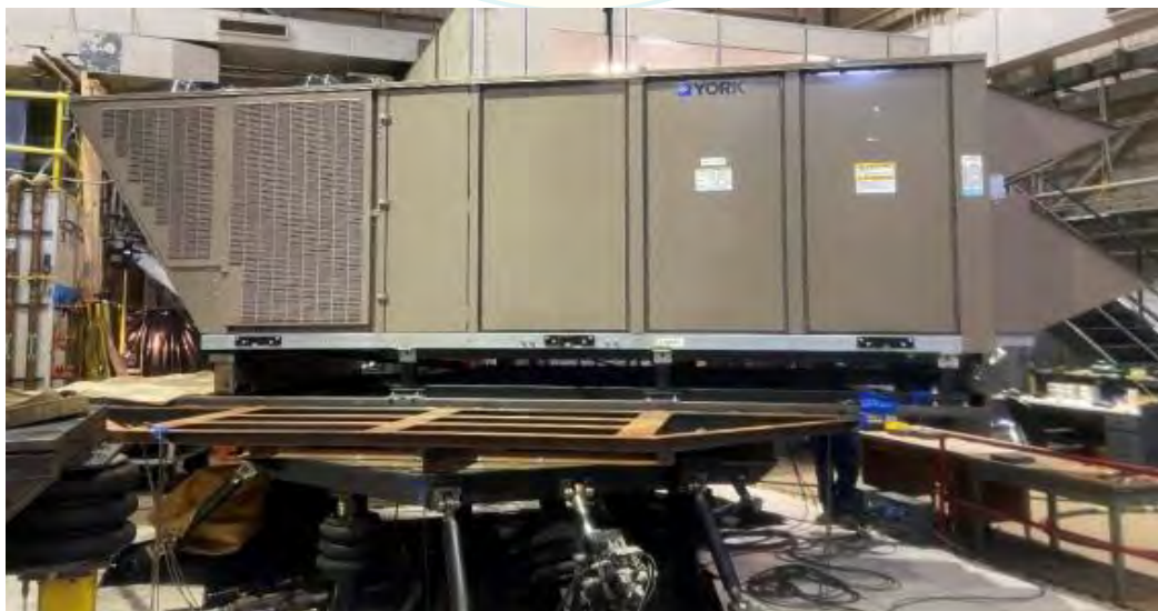
Overall view of UUT1
