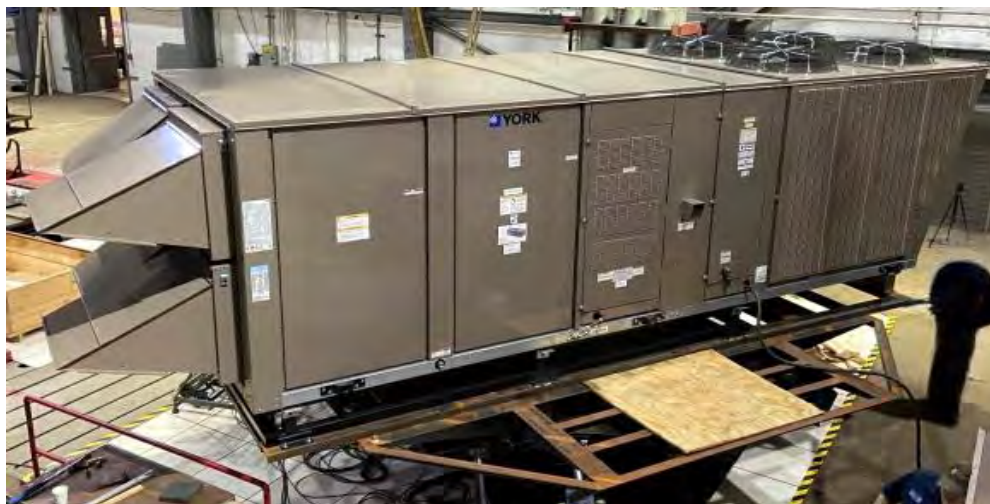
Overall view of UUT2
