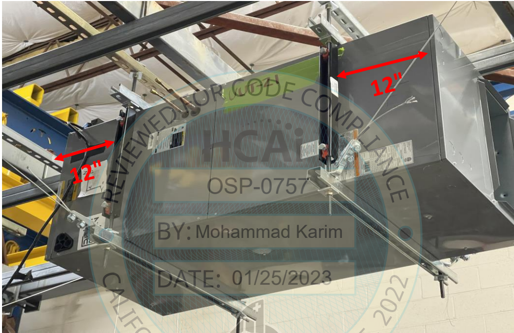
Hanging rod and cable attachment details:
