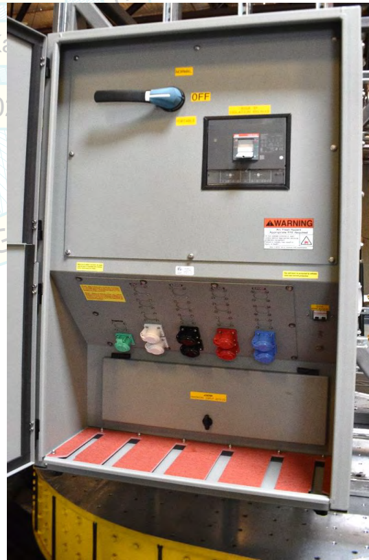
Interior view of UUT-05.
