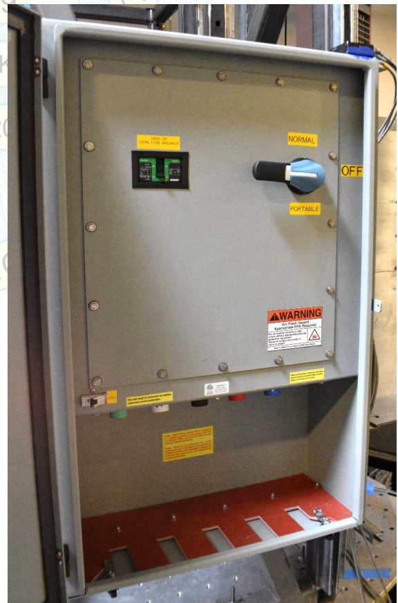
Interior view of UUT-03.
