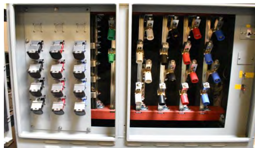
UUT-08 bottom section interior view.
