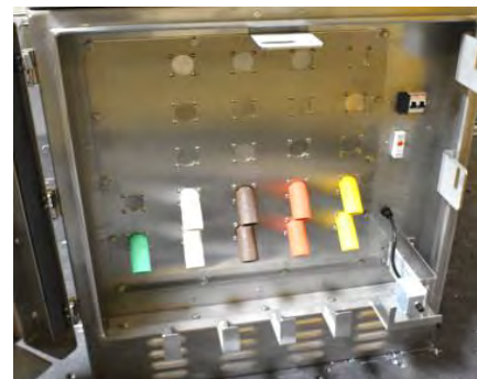
UUT-07 bottom section interior view.
