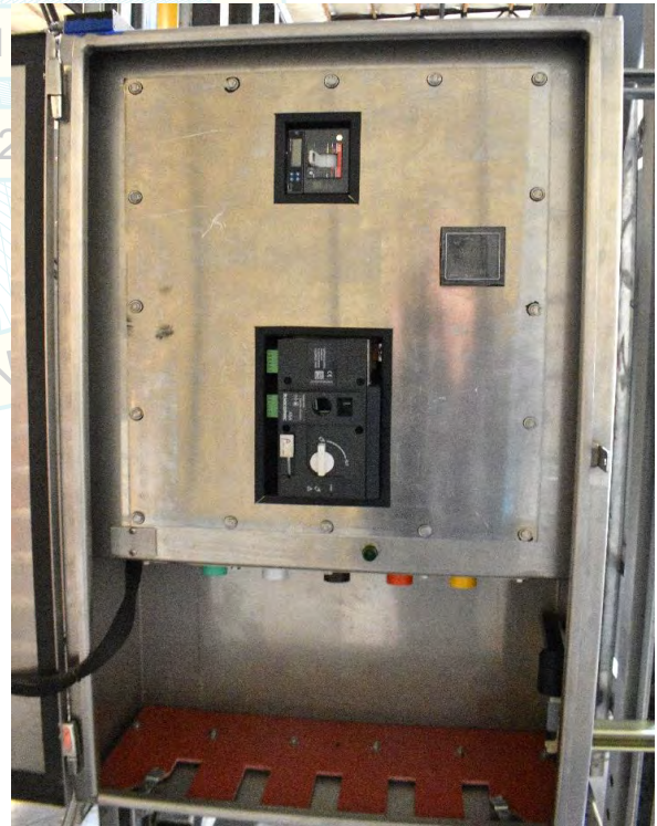
Interior view of UUT-04.
