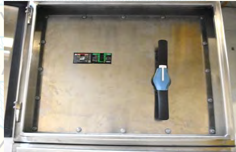
UUT-07 top section interior view.
