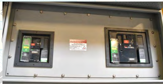
UUT-08 top section interior view.
