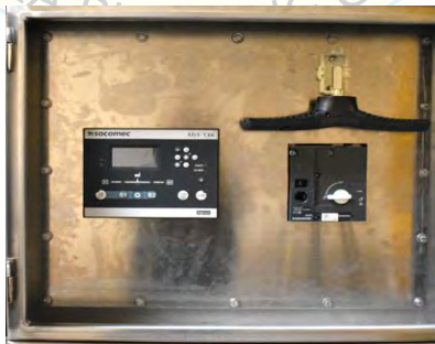
UUT-07 middle section interior view.
