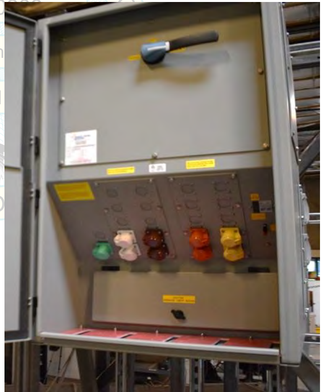
Interior view of UUT-01.
