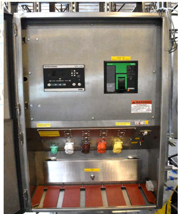
Interior view of UUT-06.
