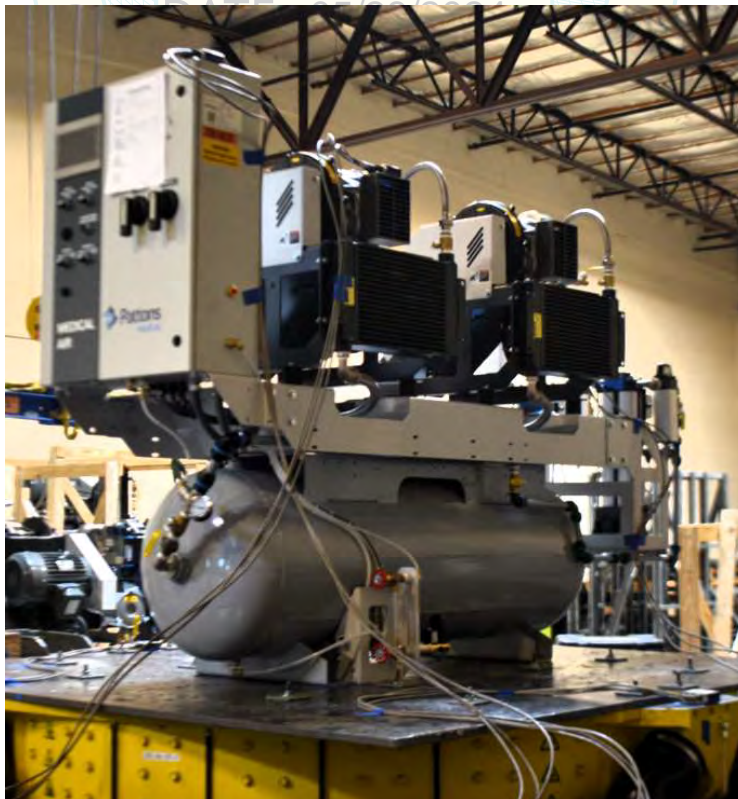
Overall Picture of UUT-01
