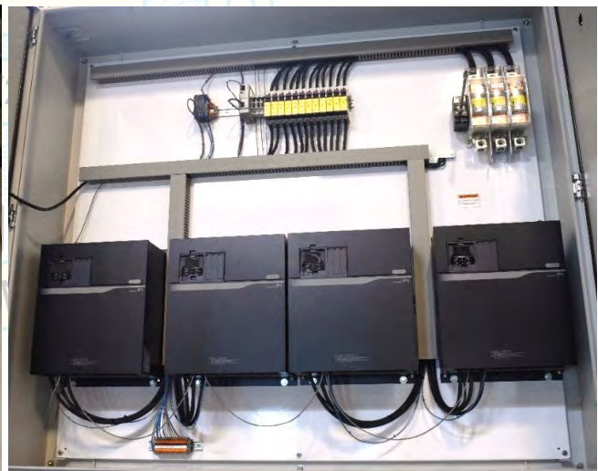
UUT-02b interior view.
