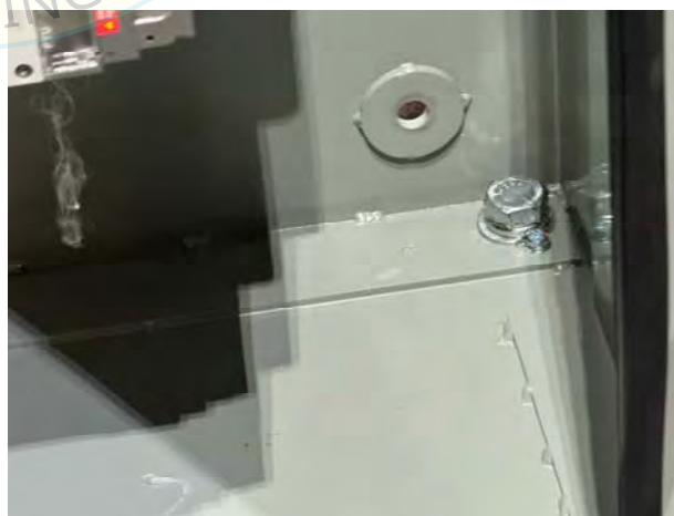
Interior of UUT9
