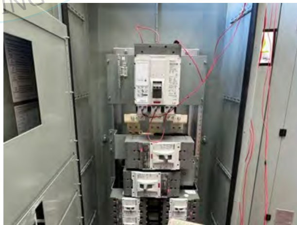
Interior of UUT3
