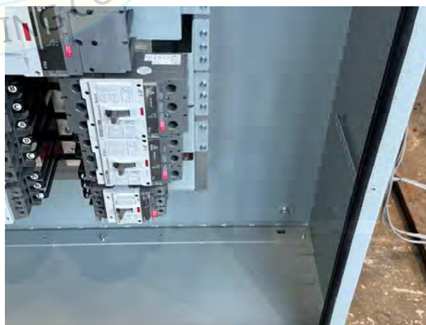
Interior of UUT4
