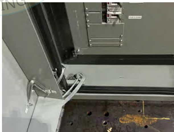
Interior of UUT8
