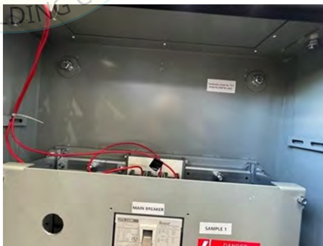
Interior of UUT1
