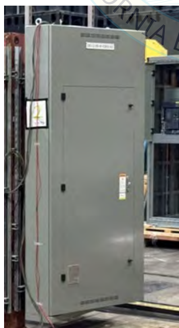
UUT2 mounted on the shake table
