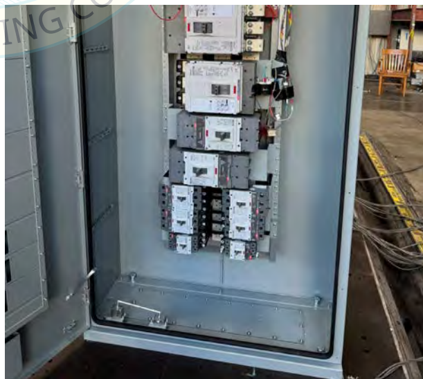
Interior of UUT5
