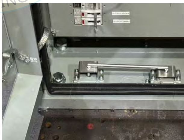
Interior of UUT7
