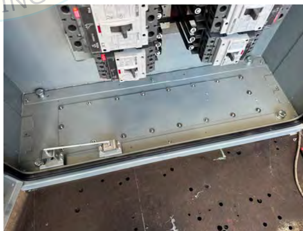
Interior of UUT6
