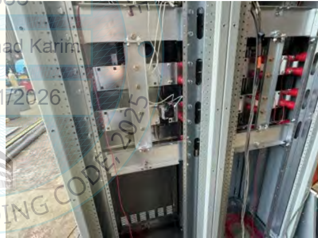
Interior of UUT1
