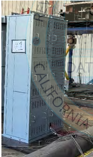
Exterior of UUT1
