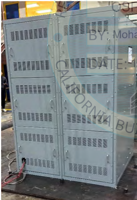
Exterior of UUT3
