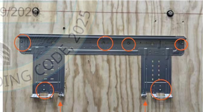
(2) Two 1/8" - 0.6" flat head set screws provided in Carrier mounting kit with
