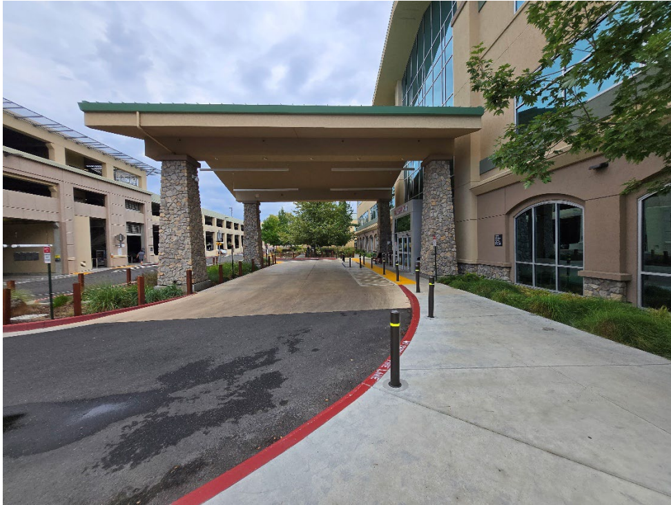
Figure 1. Example of Porte-Cochere with required sprinklers.
