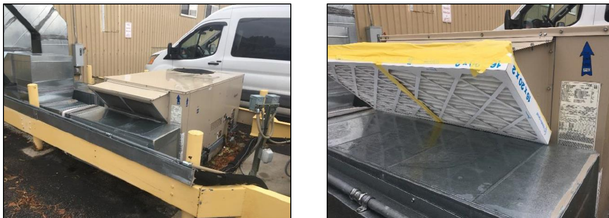
Figure 7.4 – Filtration Added to Air Intake
