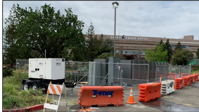
Figure 11.4 – Temporary Service Yard
