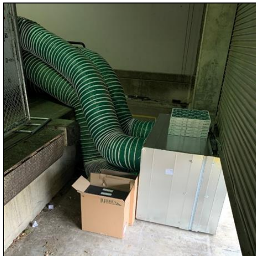
Figure 11.6 – Routing of Temporary Ventilation and Exhaust Ducts
