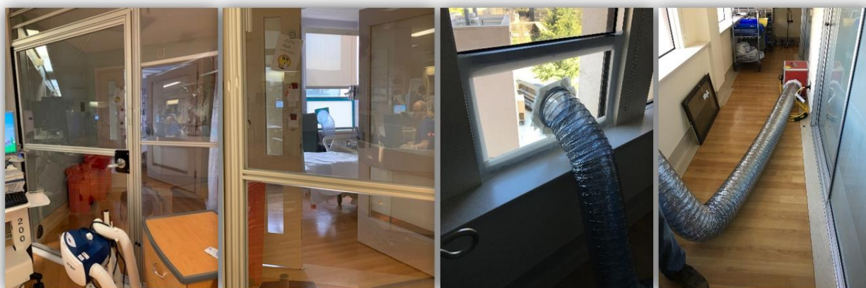
Figure 3.4 – Temporary Ducting to Outside
