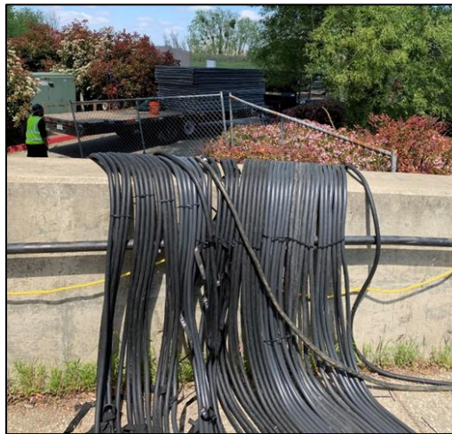
Figure 11.5 – Routing of Temporary Electrical Utilities
