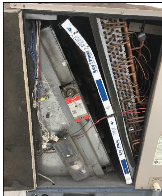
Figure 7.6 – Filter Not Seated Correctly
