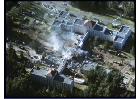
Results of the 1971 Sylmar Earthquake On Hospital Buildings
