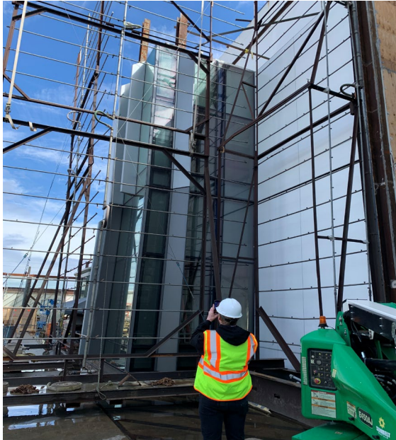
Curtain wall performance mockup
