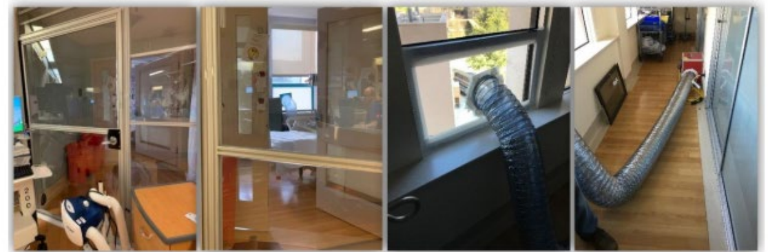
Figure 3.4 – Temporary Ducting to Outside
