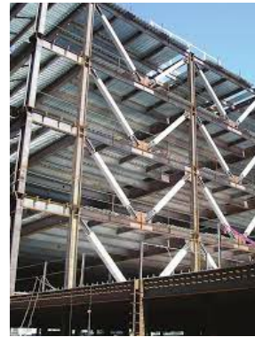
Steel Braced Frame
