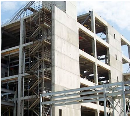
Concrete Shear wall
