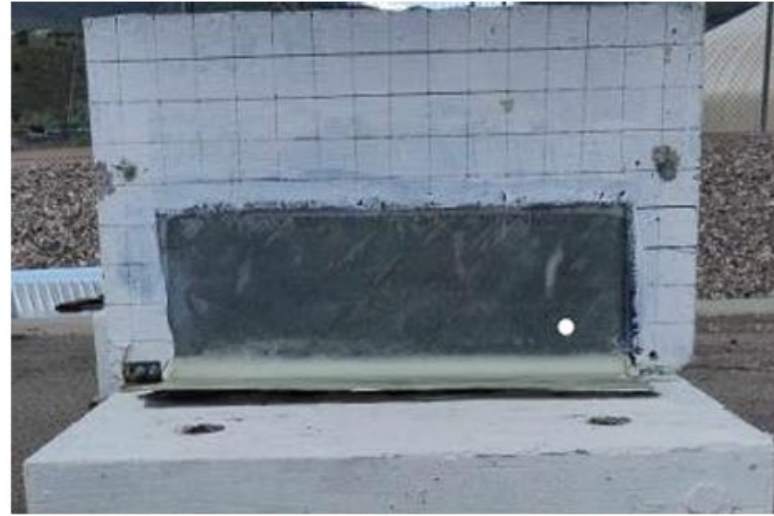
b. Debonding failure of glass fabric SP10
