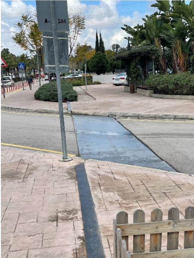
Adana City Hospital Sidewalk crosses the moat cover
