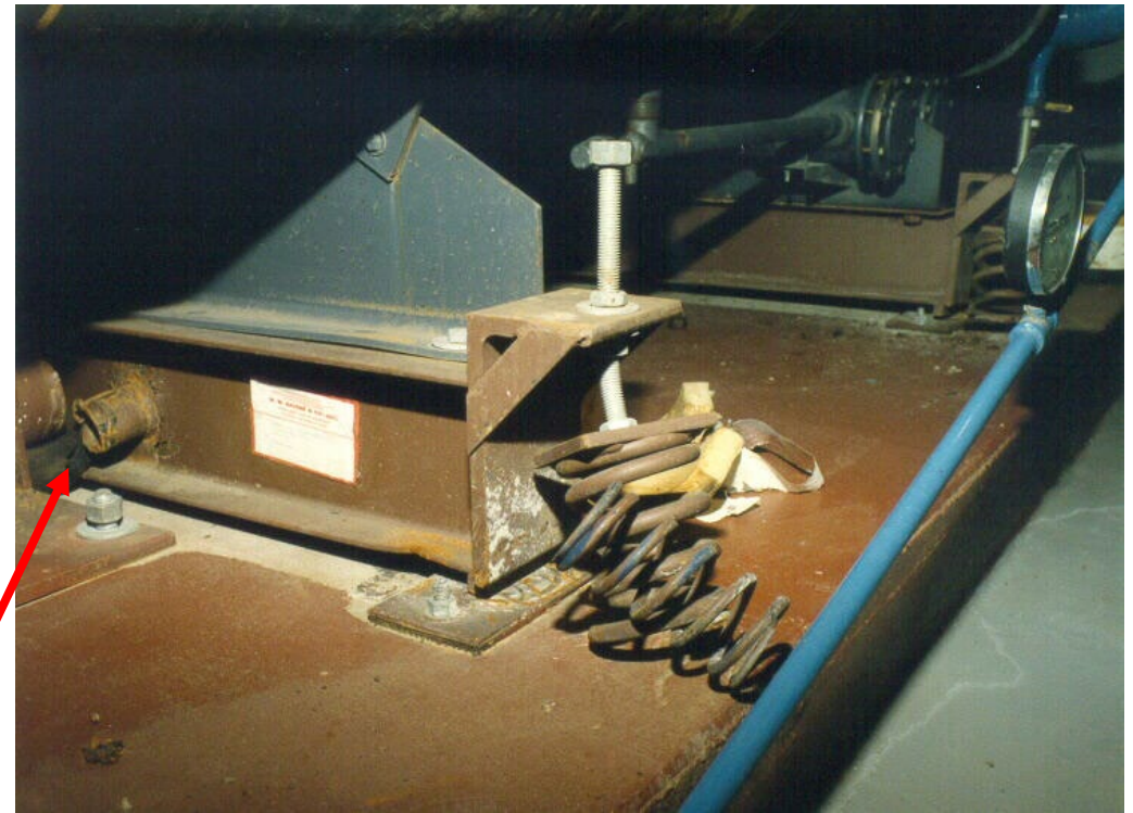
Pipe Separation from Outer Pipe Restraint
