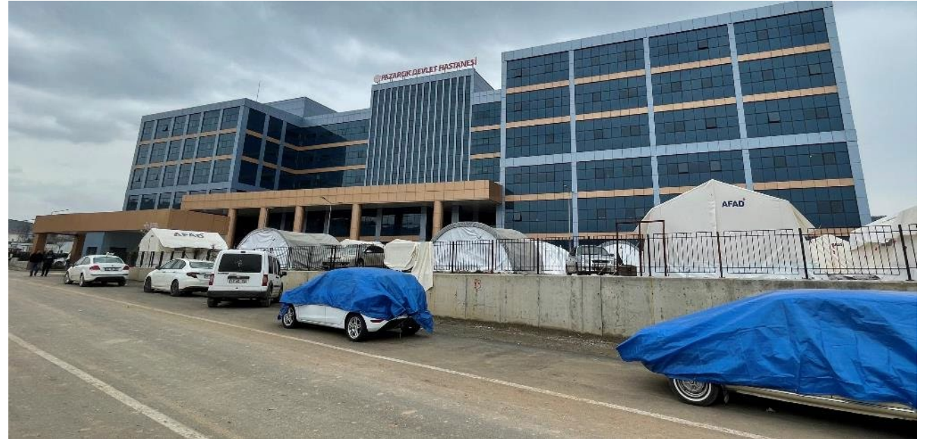
Pazarcik Government Hospital RC shear wall on 550 piles Separated by seismic joints into 5 structures PGA: 2.38 g (under review) PGV: 94 cm/s
