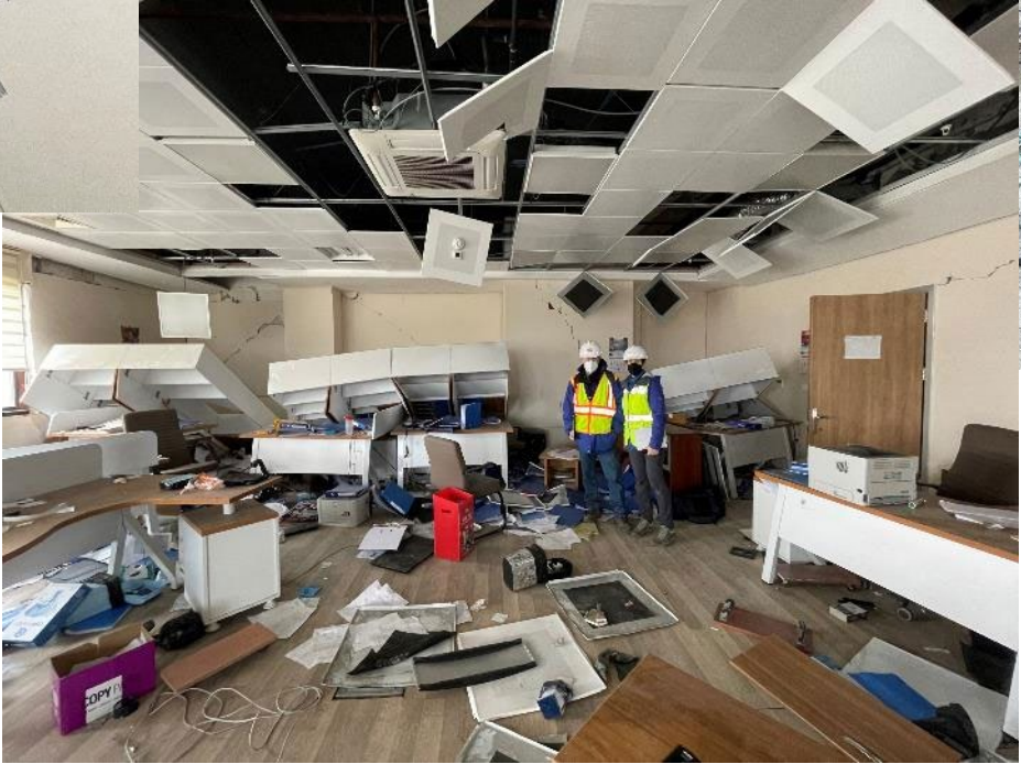
Nurdagi Government Hospital Structural and nonstructural damage
