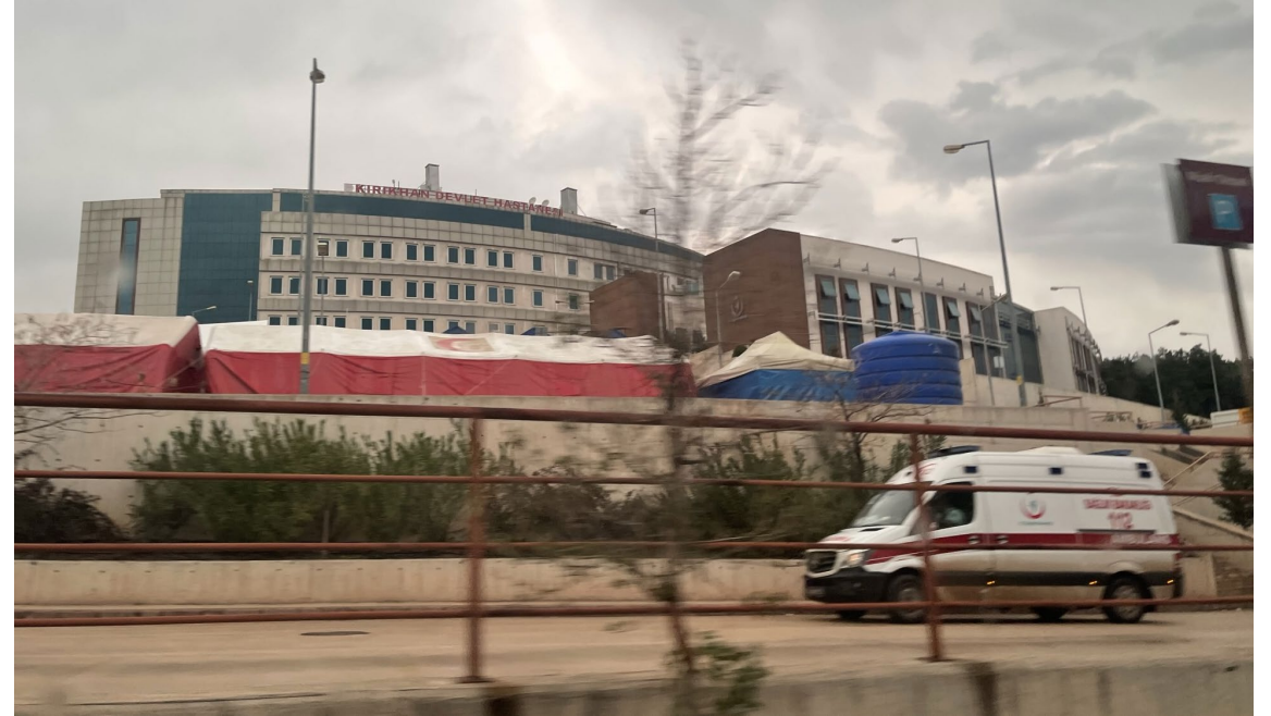
Kirikhan Government Hospital (Kirikhan Devlet Hastanesi) Built 2019
