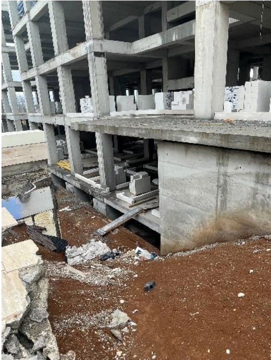
Kahramanmaraş Necip Fazıl Hospital Under Construction
