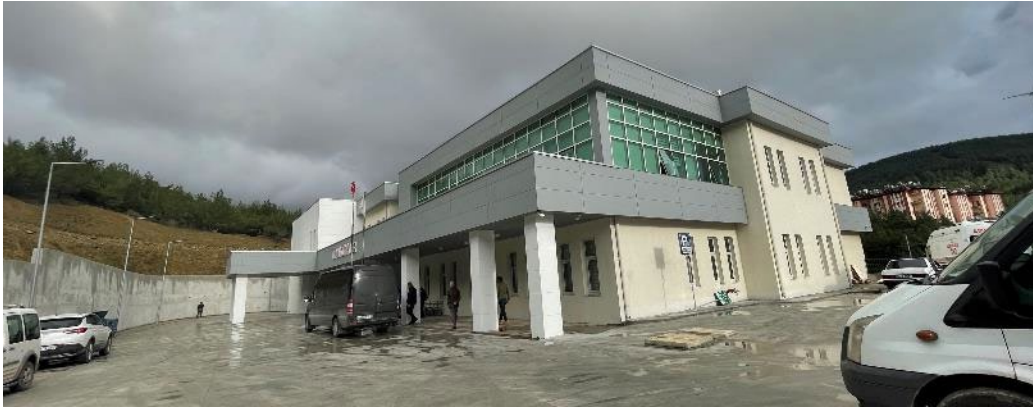
Belen Government Hospital RC shear wall PGA: 0.46 g PGV: 55cm/s
