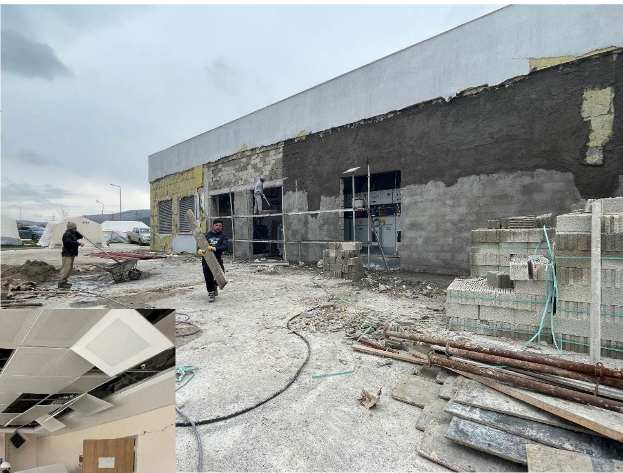
Pazarcik Government Hospital Rebuilding Central Utility Plant with same infill approach
