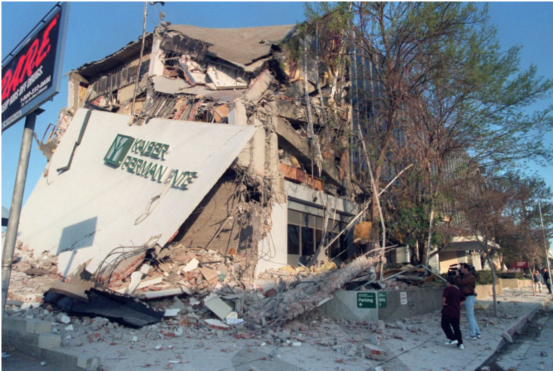
Figure 5. Damage to the Kaiser Permanente clinic building in Granada Hills during the 1994 Northridge earthquake 5
