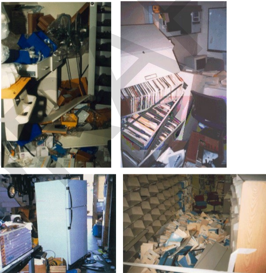
Figure 10. Examples of nonstructural damage at Olive View Hospital in the 1994 Northridge earthquake. 8
