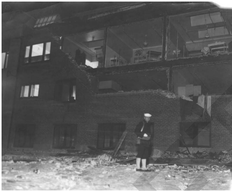
Figure 3. Damage to the Seaside Hospital during the 1933 Long Beach earthquake 3
