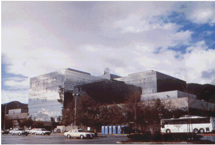
Figure 9. An outside view of Olive View Hospital Building the day after the 1994 Northridge earthquake. 8
