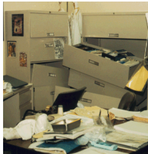
Figure 14. Instrumentation indicates overturning of file cabinets on the 6 th floor of the Olive View Hospital following the 1994 Northridge earthquake using a relevant and readily available FEMA-P58 fragility function 9 .
