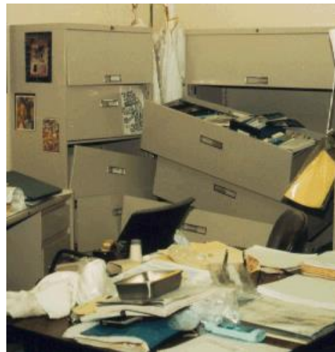
Figure 16. Instrumentation indicates overturning of file cabinets on the 6 th floor of the new Sylmar County Hospital following the 1994 Northridge earthquake using a relevant and readily available FEMA-P58 fragility function 13 .
