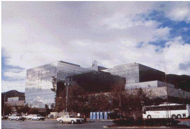
Figure 10. An outside view of the new Sylmar County Hospital Building (now Olive View-UCLA Medical Center) the day after the 1994 Northridge earthquake. 10
