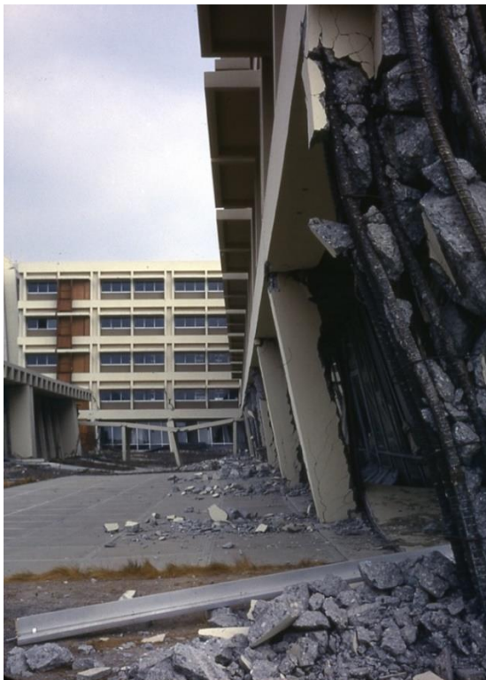
Figure 4. Damage to the original Olive View Hospital during the 1971 San Fernando earthquake 4 ; this facility was demolished and replaced by a new hospital building.
