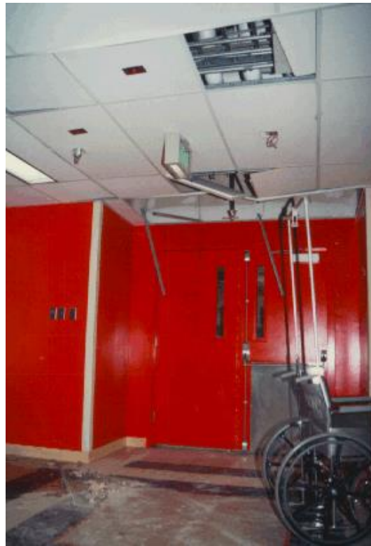
Figure 15. Instrumentation indicates displaced suspended ceiling tiles on the first floor of the new Sylmar County Hospital following the 1994 Northridge earthquake using a relevant and readily available FEMA-P58 fragility function 13 .
