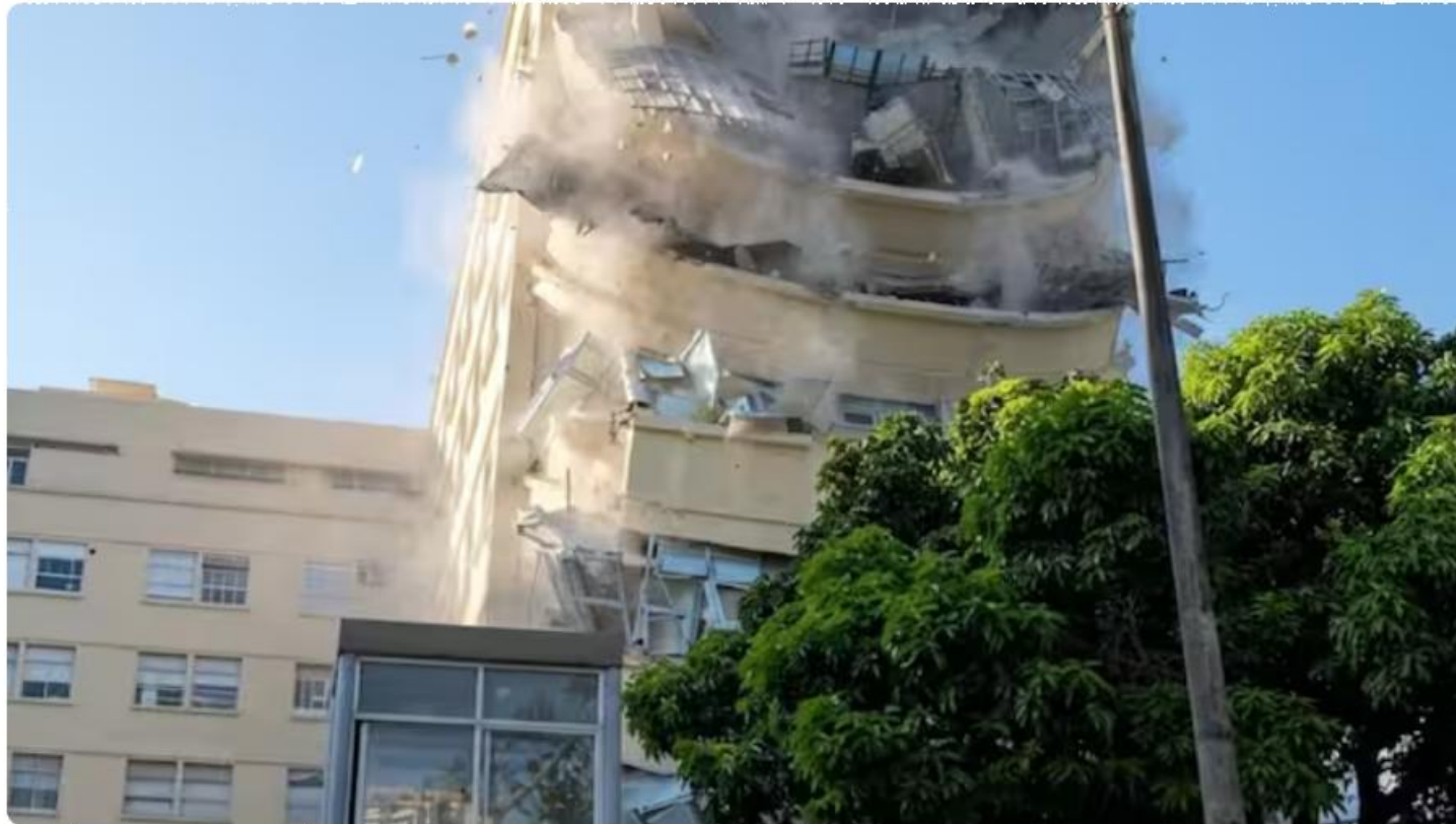
Three floors of the Hospital Universitario del Valle in Cali collapsed after a powerful 7.4-magnitude earthquake struck western Colombia (Image/X)
