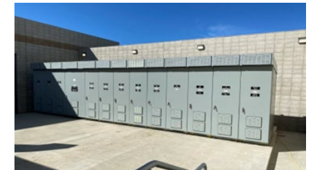
Campus Main Service/ Microgrid Gear
