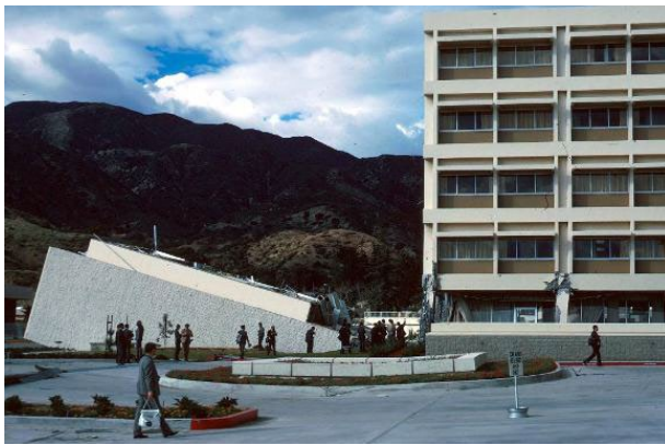
Figure 2. The 1971 San Fernando earthquake resulted in partly detached staircase and severely damaged buildings at the Olive View Hospital. (Source: USGS earthquake photo archive, available online at https://library.usgs.gov/photo/#/?category1=earthquakes&collection2=san%20fernando%20earthquake,%20february%201971 )
