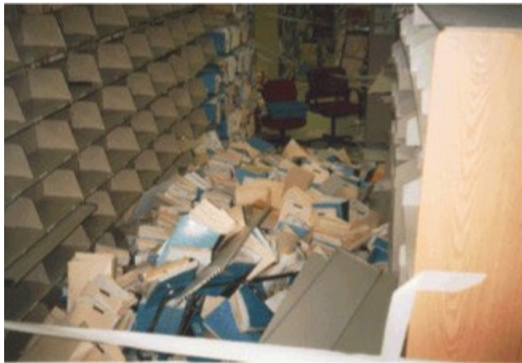
Figure 2. Examples of nonstructural damage at Sylmar County Hospital in the 1994 Northridge earthquake (Naeim 1997)
