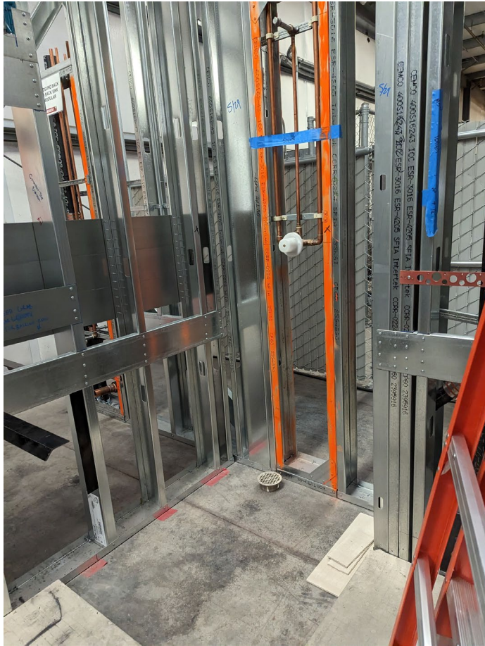
ICU Room Shower
