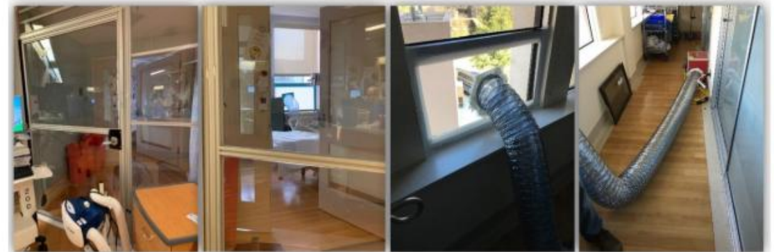
Figure 3.4 – Temporary Ducting to Outside
