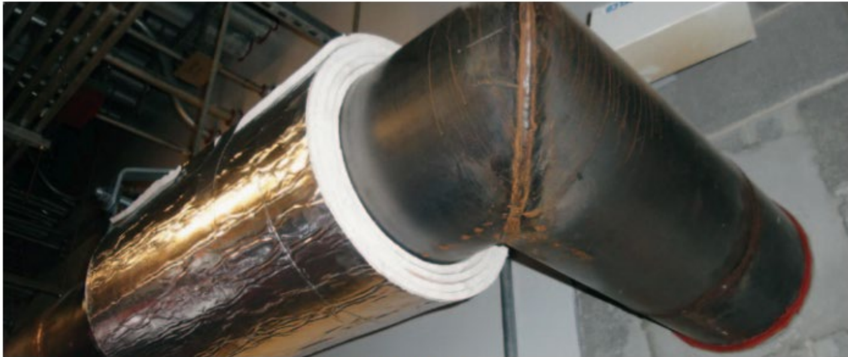
Fire-resistant pipe-protection system during installation on horizontal offset fuel pipe.
