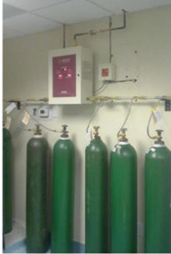
Figure 3 Cylinder Manifold – Make Sure to Restrain Tank
