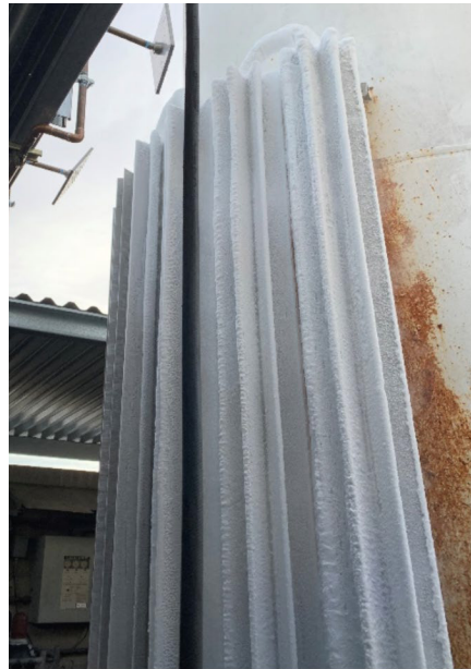
Figure 8 Do Not Mount Evaporator Too Close to Other Objects that May Prevent Air Circulation
