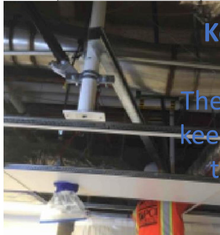
Typical STANDARD P FINIS Typical pendant and brace installation configuration
