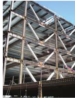
Steel Braced Frame
