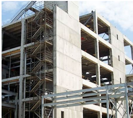
Concrete Shear wall
