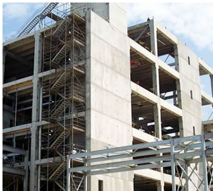
Concrete Shear wall
