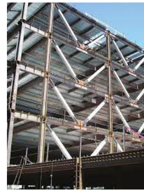
Steel Braced Frame
