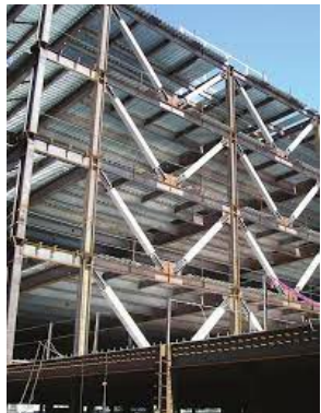
Steel Braced Frame
