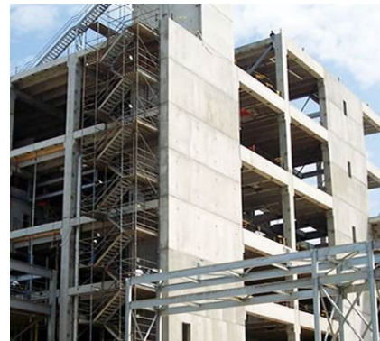
Concrete Shear wall
