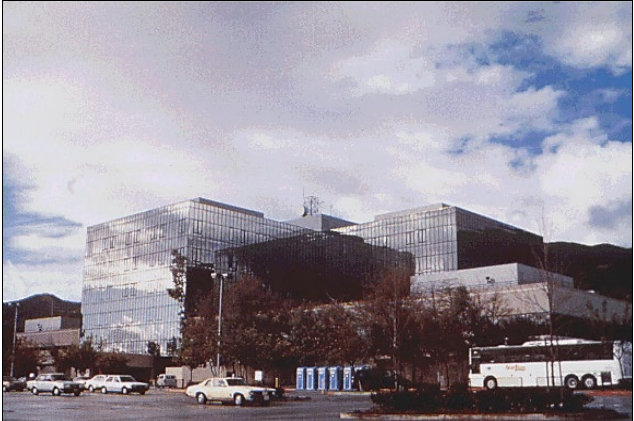
Figure 10. An outside view of the new Sylmar County Hospital Building (now Olive View-UCLA Medical Center) the day after the 1994 Northridge earthquake. 11
