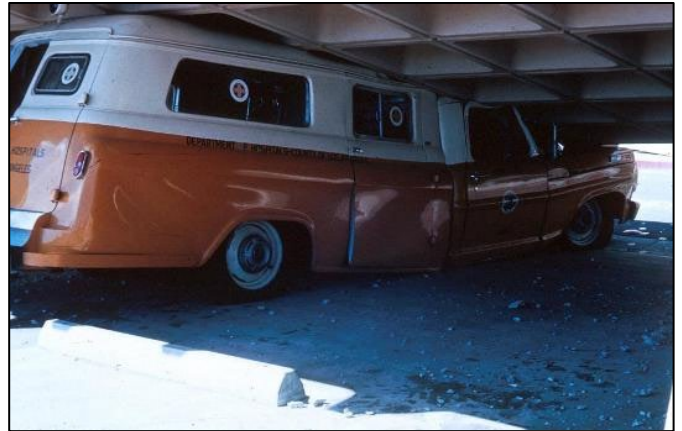
Figure 4. Damage to the original Olive View Hospital during the 1971 San Fernando earthquake; this facility was demolished and replaced by a new hospital building. 4
