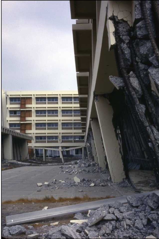
Figure 4. Damage to the original Olive View Hospital during the 1971 San Fernando earthquake; this facility was demolished and replaced by a new hospital building. 4
