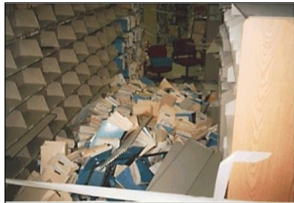
Figure 11. Examples of nonstructural damage at the new Sylmar County Hospital during the 1994 Northridge earthquake. 12
