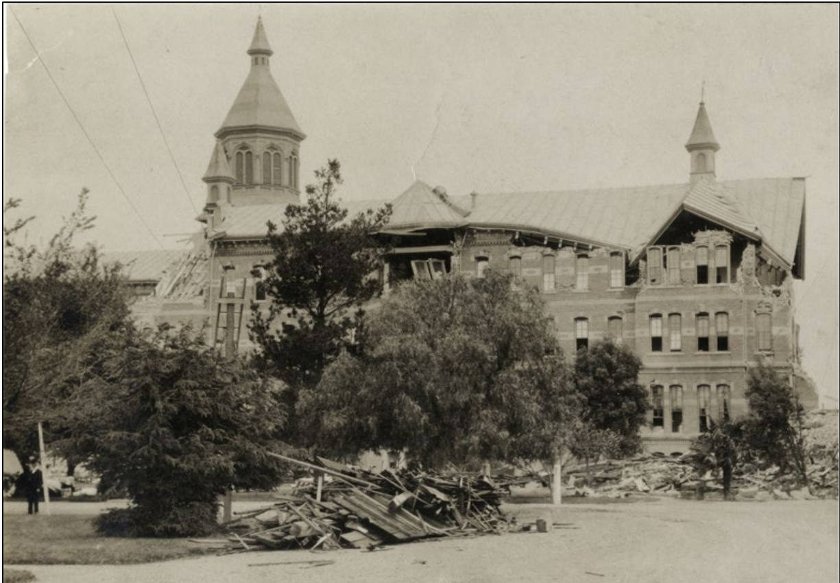
Figure 1. Damage to the San Jose Agnew Mental institution during the 1906 San Francisco earthquake. 1
