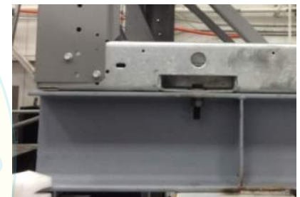
Bolted base connection
