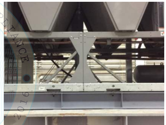
Bolted base connection with neoprene pad
