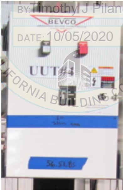
UUT4 was mounted to the wall fixture with (4) 1/4" diameter grade 5 bolts, washers and nuts. The mounting locations were spaced approximately 22.0" heightwise and 13.0" widthwise.
