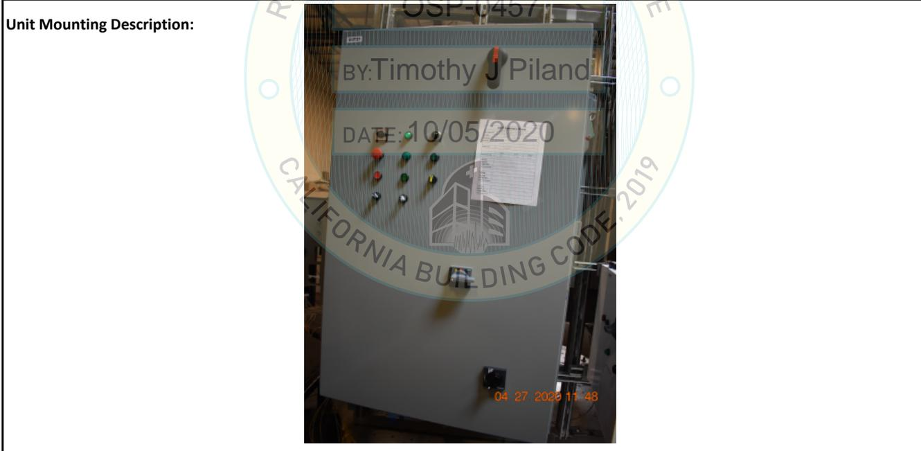
UUT26 was mounted using (4) 3/8" diameter grade 5 bolts, circular washers, 3"x3"x3/8" carbon steel plate washers and channel nuts through a welded bracket onto the wall fixture. The bolts were spaced 61.5" heightwise and 30.0" widthwise.
