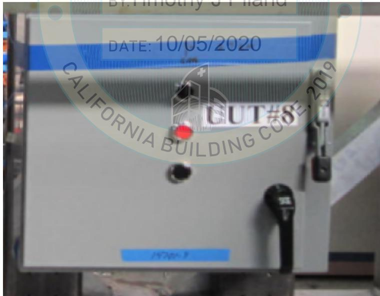
UUT8 was mounted to the wall fixture with (4) 1/2" diameter grade 5 bolts, washers and nuts. The mounting locations were spaced approximately 18.0" heightwise and 19.0" widthwise.
