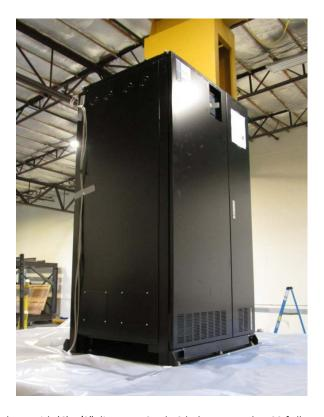
The unit was rigidly mounted at its base with (6) 1/2" diameter Grade 8 bolts, torqued to 80 ft-lb.
