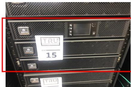
UUT 3b was mounted within a 4-Post Seismic Rack (PN: GL840EZ-3042). UUT 3b was mounted to the rack within the cabinet with a Vertiv rack slide kit (PN: RMKIT18-32). Eight (8) M5 screws and clips, provided by Great Lakes, were used to secure the UUT to the rack.
