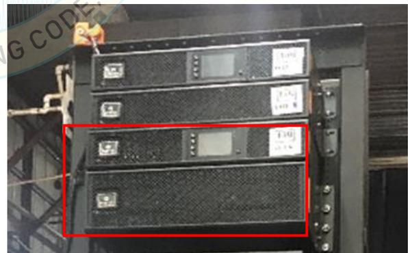
UUT 1c was mounted to a 2-Post Seismic Rack (PN: SB85219084). UUT 1c was attached to the 2-Post rack with a 4U/6U TELECOMRKIT.
