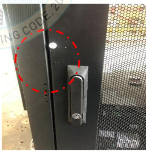
The configuration rack was mounted rigid using four (4) 5/8" - 11 Grade 8 Hex Bolts and Lock Washer and Square Washer. Unit maintained structural integrity and remained functional per manufacturer requirement. Doors sesimically modified with a #12 self tapping screw.
