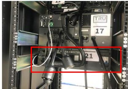
UUT 3f was mounted within a 4-Post Seismic Rack (PN: GL840EZ-3042). UUT 3f was mounted to the rack within the cabinet with a Vertiv rack slide kit (PN: RMKIT18-32). Eight (8) M5 screws and clips, provided by Great Lakes, were used to secure the UUT to the rack.
