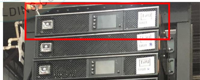
UUT 1a was mounted to a 2-Post Seismic Rack (PN: SB85219084). UUT 1a was attached to the 2-Post rack with a 2U TELECOMRKIT.
