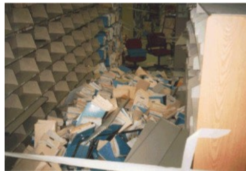
Figure 10. Examples of nonstructural damage at Olive View Hospital in the 1994 Northridge earthquake 8 .
