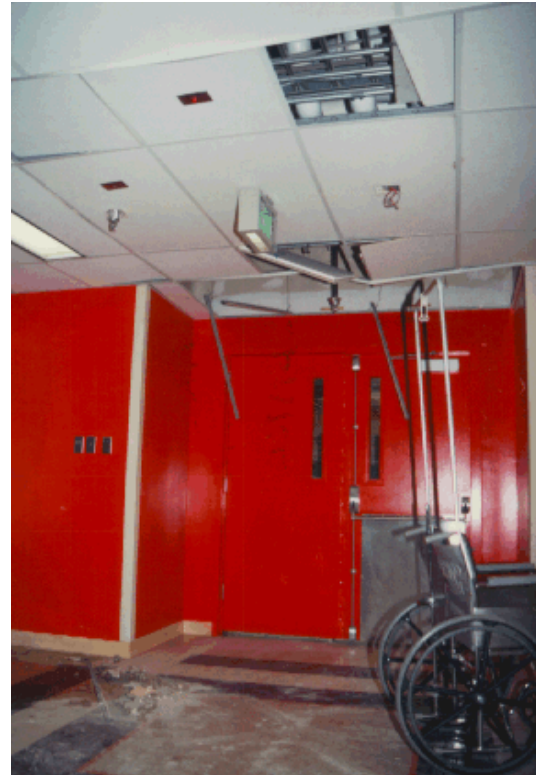
Figure 13. Instrumentation indicates displaced suspended ceiling tiles on the first floor of the Olive View Hospital following the 1994 Northridge earthquake using a relevant and readily available FEMA-P58 fragility function 9 .
