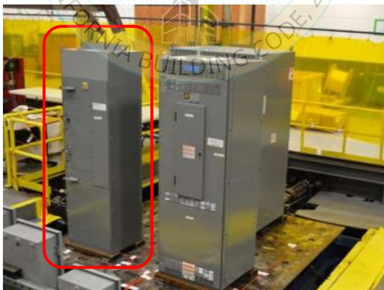
Rigid floor mount with (4) 1/2-13 grade 5 bolts and Bellville conical spring washers at 60 ft-lbs torque.
