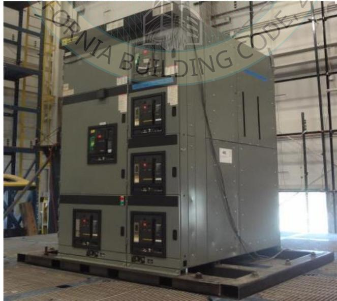
Rigid floor mount with (11) 1/2-13 grade 5 bolts and Bellville conical spring washers at 65 ft-lbs torque.
