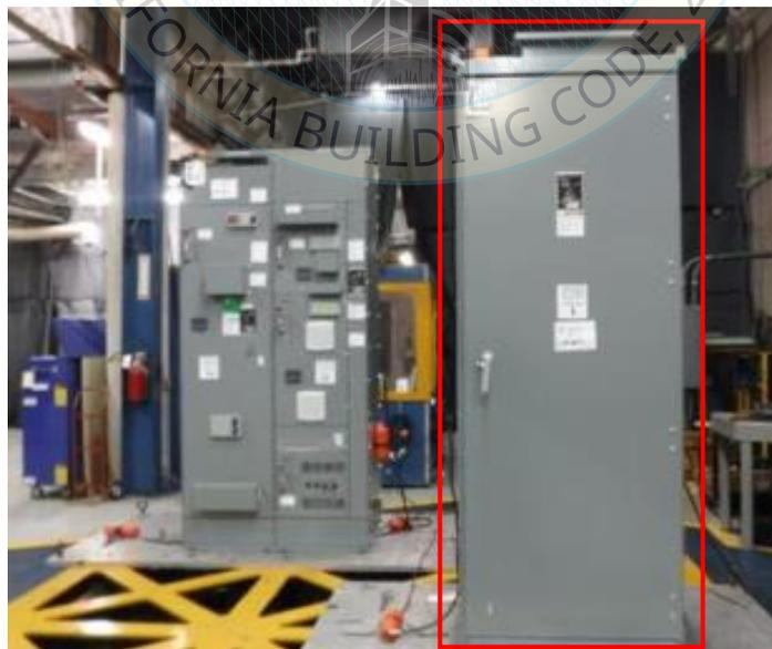
Rigid floor mount with (9) 1/2-13 grade 5 bolts and Bellville conical spring washers at 70 ft-lbs torque.
