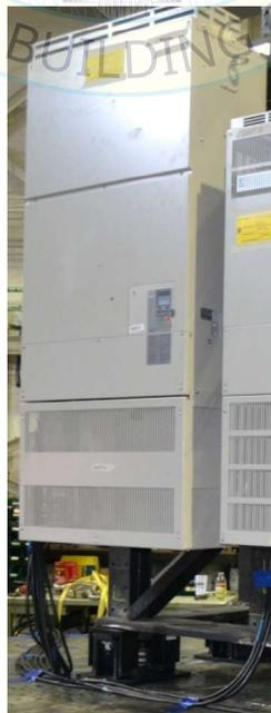
All units were filled with contents and maintained structural integrity and functionality after AC-156 test.
