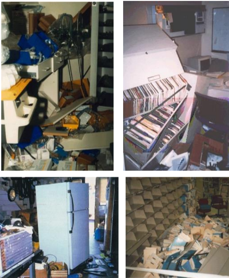
Figure 11. Examples of nonstructural damage at the new Sylmar County Hospital during the 1994 Northridge earthquake 10 .
