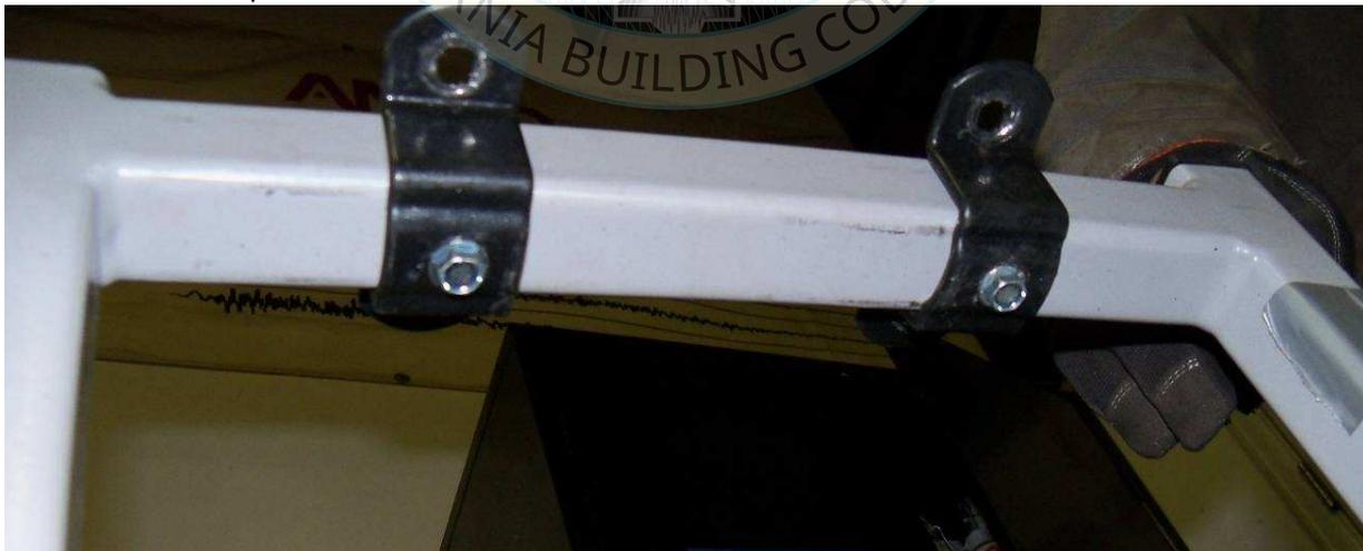
After the installation of these screws, the racks were re-tested and no slippage of the battery mounting rails was observed
