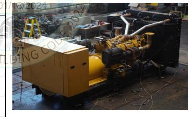
UUT10 was base mounted to test fixture using six (6) VMC M2SSH-1E 5150 spring isolators (and included hardware). Twelve (12) 3/4" Grade 8 bolts are used to mount the isolators to the test fixture. Unit maintained structural integrity and remained functional per manufacturer requirement after shake table test. Contents were included in testing per operating conditions.
